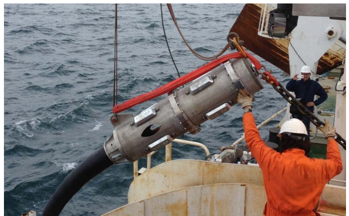
▲ MacArtney ILT deployed to connect multiple tidal turbines within an offshore tidal farm, to a central power conditioning unit (image courtesy of EDF).
