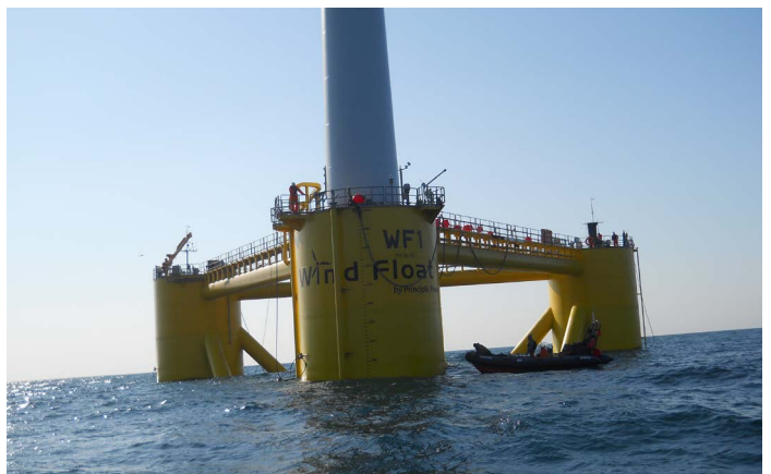
▲ The prototype WindFloat (floating wind turbine) moored offshore Portugal. The scope of MacArtney supply included an InLine Termination, hang-off clamps, bend stiffeners, distributed buoyancy modules, general cable protection equipment, termination of dynamic medium voltage umbilical and retrofitting of a water blocking device.
