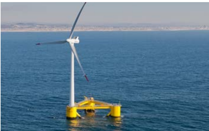
▲ The prototype WindFloat (floating wind turbine) moored offshore Portugal. The scope of MacArtney supply included an InLine Termination, hang-off clamps, bend stiffeners, distributed buoyancy modules, general cable protection equipment, termination of dynamic medium voltage umbilical and retrofitting of a water blocking device.
